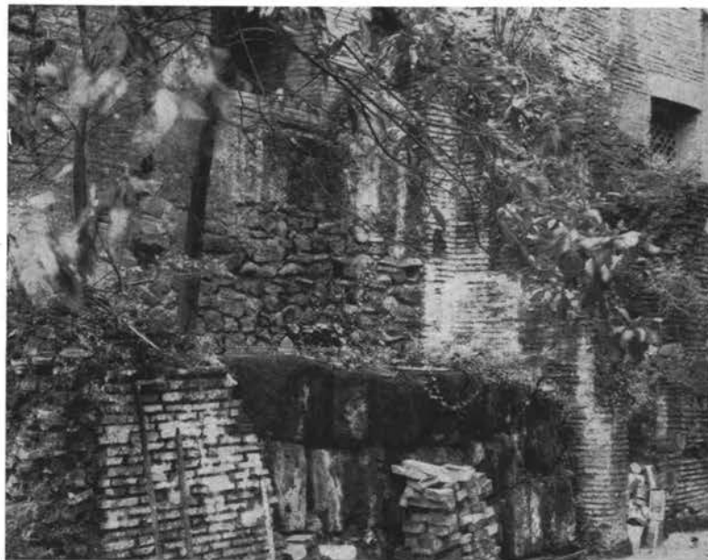
Fig. 105. S. Martino ai Monti, Roman Hall, ninth century foundations sealing the entrance into D; exterior
